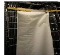
Use of Flame Retardant Plastic Sheeting as a Barrier
