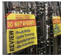
Rear Panel Barriers Using Velcro Straps To Secure
