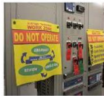
Front Panel Barriers Using Magnets To Secure
